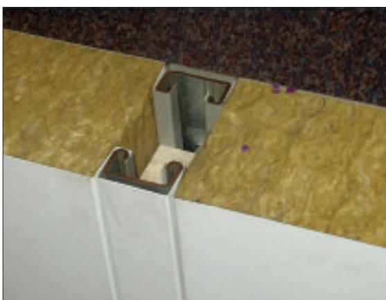
Figure 17: Insulated core panels – internal panel
