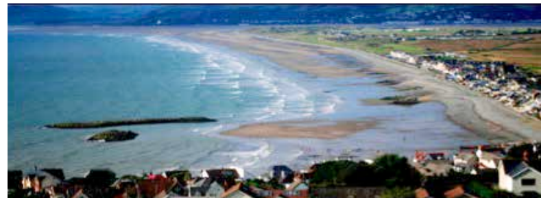
The alteration of the beach, evident from a photograph of the sand extrusion at South Borth. A sand bar extrudes to the sea in the lee of the offshore structure
